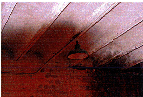
Left - F.F.D 1 – The roof structure in the personnel de-contamination and changing room indicating the roof beams with 'U' section facing down in the non splinter proof construction method © by Graham Smith 2010
