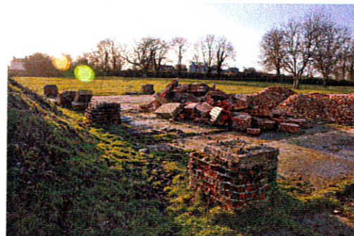
Kimbolton – Remnants of brick bases from the unloading gantries 2No the remnants of the train line can be seen between the first pair. © by Graham Smith 2010
