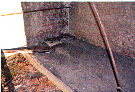
Left : The brick 1 st floor building of one of the charging buildings that housed the vesicant prior to charging into the weapons showing the 3 No pipe holes feeding through to the charging equipment below. . © by Graham Smith 2010
