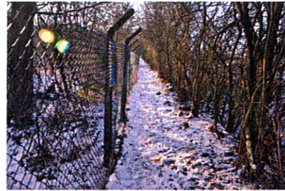
Right – Picture taken outside of the Coppice Wood perimeter fence showing the 1.5-2.0m clearance of vegetation to allow the fence to be checked. © by Graham Smith 2010
