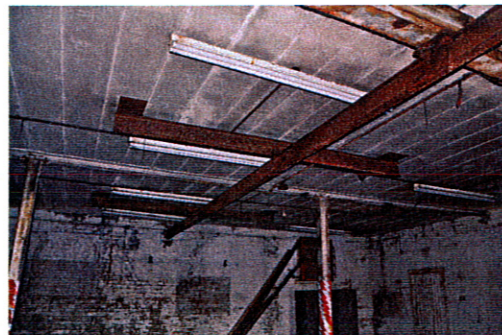
Left - F.F.D 1 – The roof structure in the personnel de-contamination and changing room indicating the roof beams with 'U' section facing down in the non splinter proof construction method © by Graham Smith 2010
