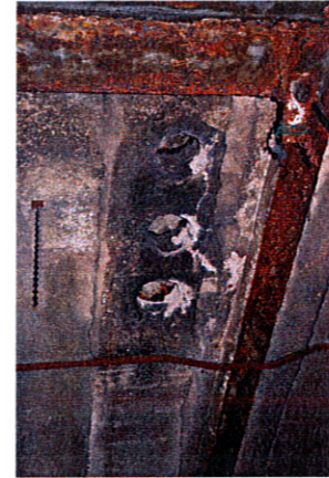
Left : The brick 1 st floor building of one of the charging buildings that housed the vesicant prior to charging into the weapons showing the 3 No pipe holes feeding through to the charging equipment below. . © by Graham Smith 2010
