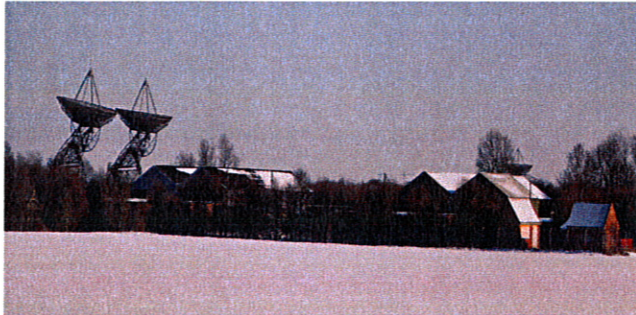
F.F.D 4 Lords Bridge – Viewed from the south looking North East, the two bays of the building on the left is the roof of the empty storage building whilst the two on the right are of the bonding building, the small building on the far right is new and to the far left are two of the MRAO radio telescopes. © Graham Smith 2009
