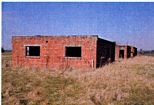
F.F.F 5 – Remains of the office building in the foreground followed by the toxic & non toxic mess and then the decontamination & changing room block – © Graham Smith 2010
